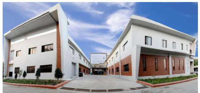
Tempsens Instruments U# II Cable Plant
